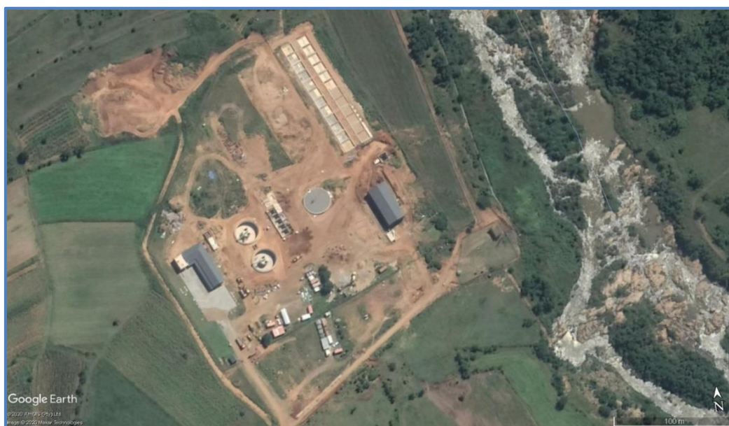
Figure 17.75 Construction of new 15 Mℓ/day WTP at Frischgewaagd along the Phongola River (Google Earth 2020: website).
