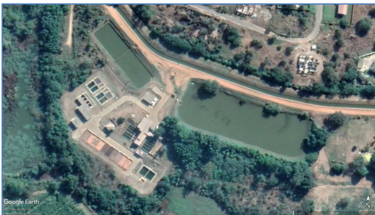
Figure 17.59 Aerial view of Phongola Water Treatment Plant
