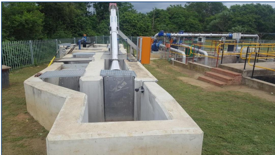
**Figure 19.21** Lynnfield Park WWW head of works showing manual and mechanical screening channels.
