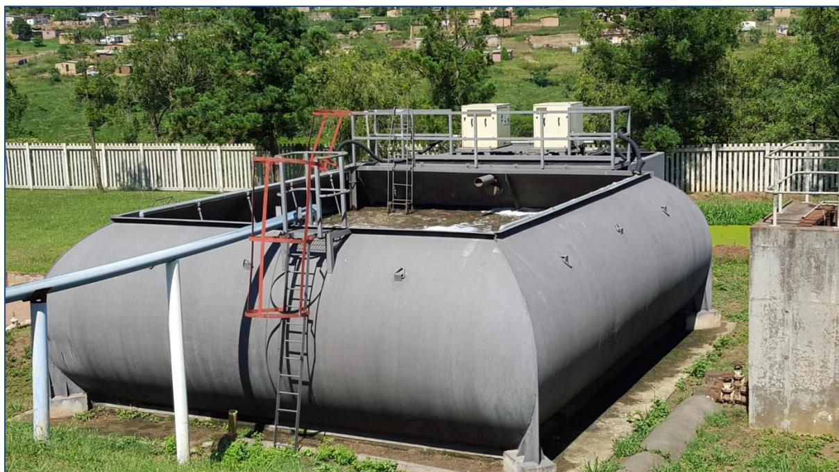
**Figure 19.12** Sequencing Batch Reactor (SBR) Albert Falls North WWWW.
