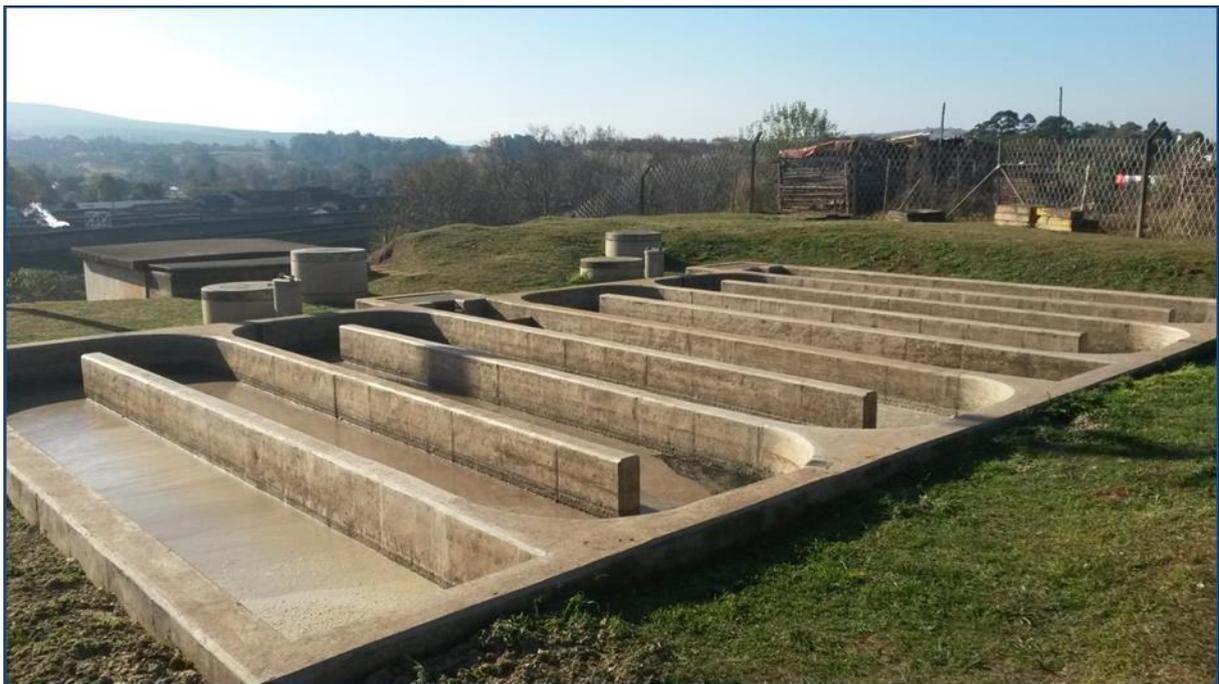
**Figure 19.14** Howick WWW Chlorine Contact Tank.
