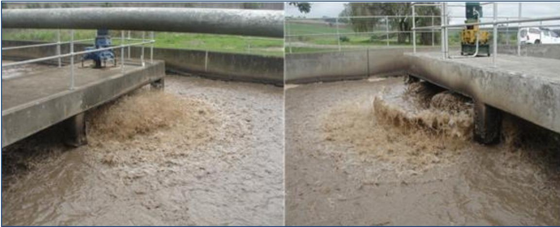
**Figure 19.30** Different Mechanical Surface Aerators in Cool Air Reactor 1 and 2.
