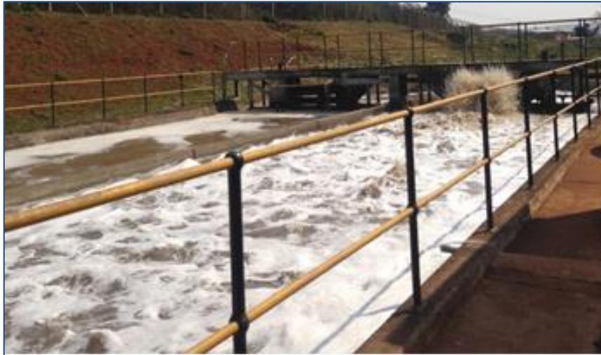
**Figure 19.27 Appelsbosch WWT Oxidation Ditch (Aeration Tank).**
