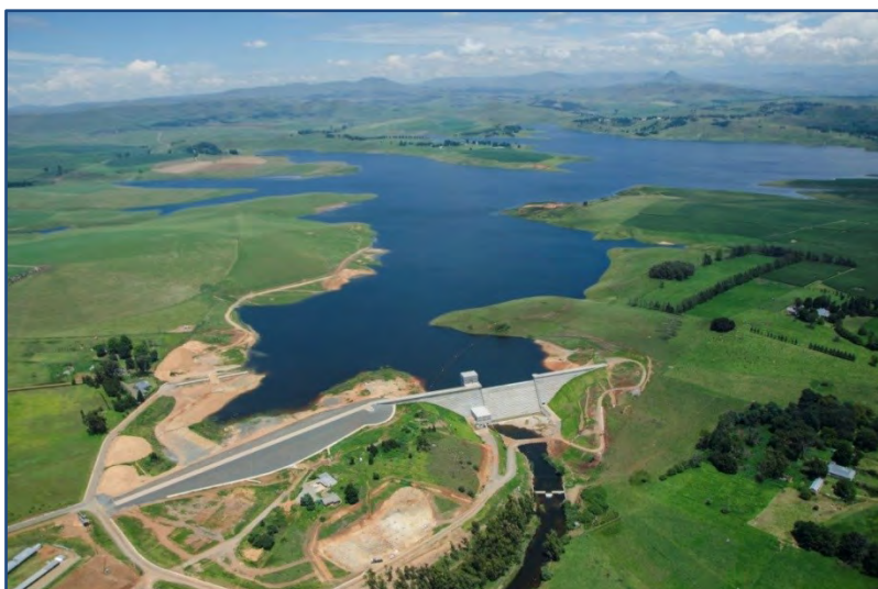
Figure 7.23 Spring Grove Dam.
