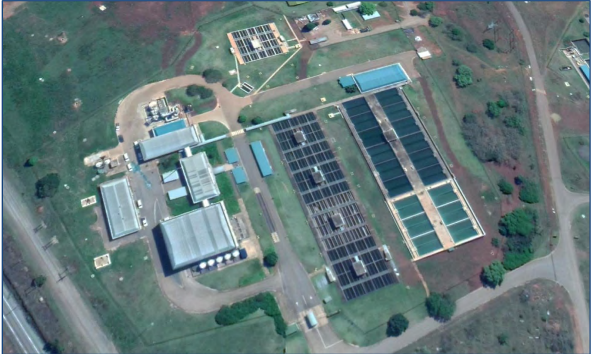
Figure 7.28 Midmar Water Treatment Plant after the upgrade.
