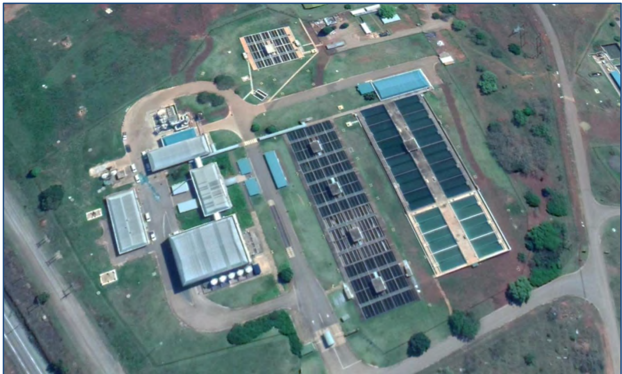
Figure 7.28 Midmar Water Treatment Plant after the upgrade.
