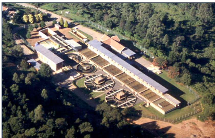
Figure 7.35 D.V. Harris Water Treatment Plant.
