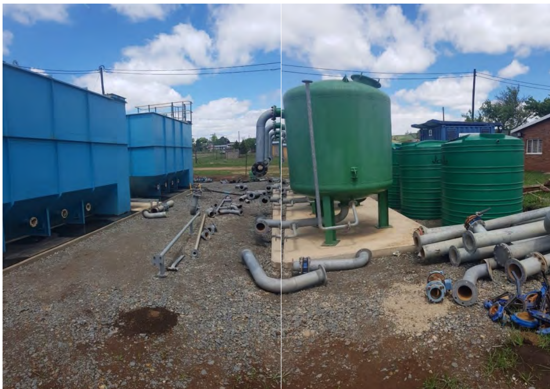
Figure 7.78 1 Ml/day being constructed at the Lidgetton System.
