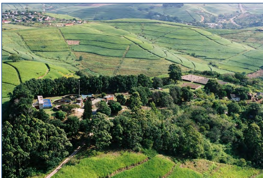
Figure 11.25 Umzinto Water Treatment Plant.
