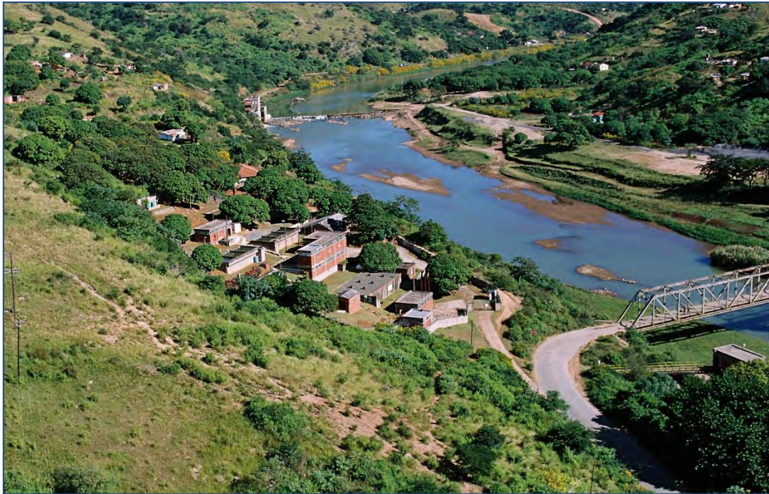
Figure 11.24 Craigieburn Water Treatment Plant (decommissioned).
