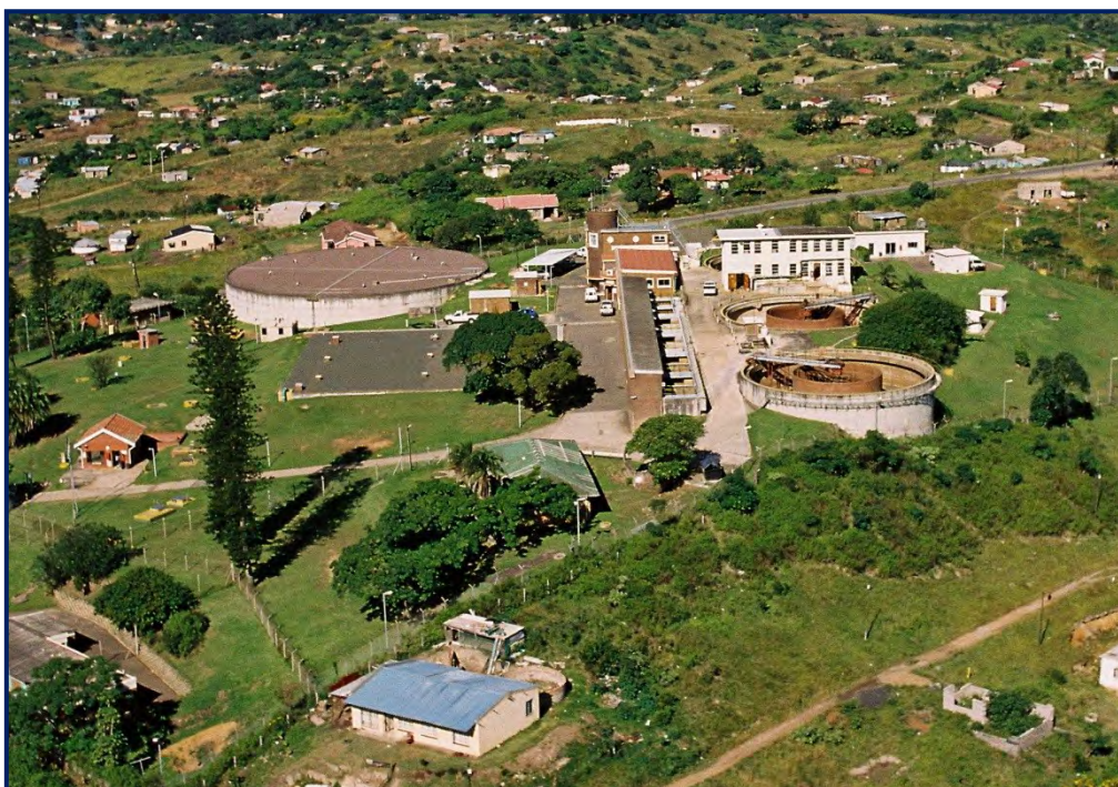
Figure 11.22 Amanzimtoti Water Treatment Plant.
