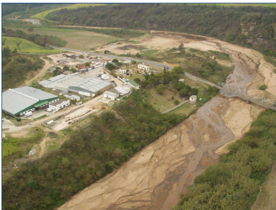
Figure 11.27 Mtwalume Water Treatment Plant.
