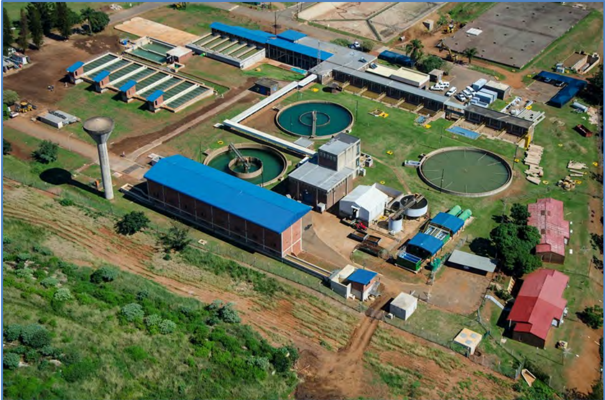
Figure 12.17 Hazelmere Water Treatment Plant.
