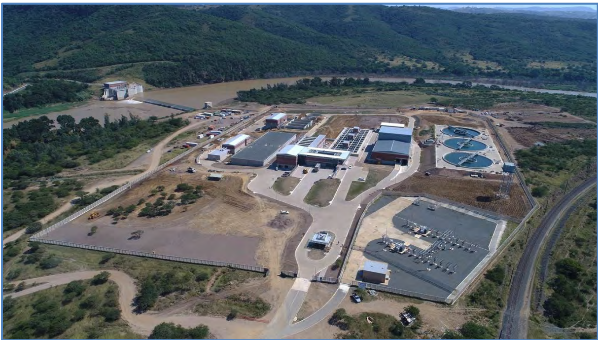
Figure 12.20 Lower Thukela Water Treatment Plant
