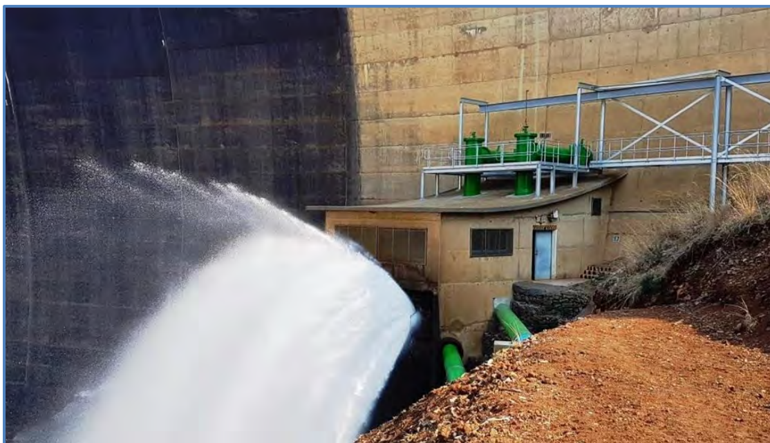
Figure 12.53 Abstraction point (Craigie Burn Dam)
