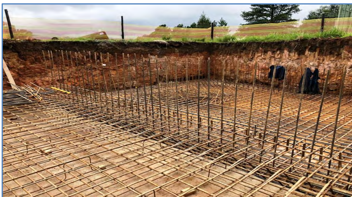
Figure 12.54 Transfer Pump Station in Construction (Late 2019)
