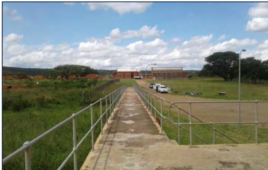
Figure 13.36 Olifantskop Water Treatment Plant (unknown date).
