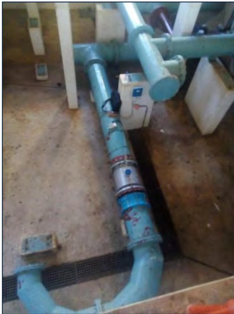
Figure 13.45 Ekuvukeni sales meter (Umgeni Water 2019).
