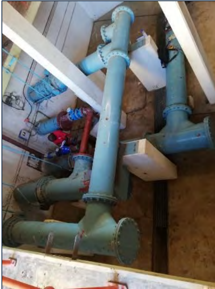
Figure 13.46 Waaihoek and Mabhekazi sales meters (Umgeni Water 2019).
