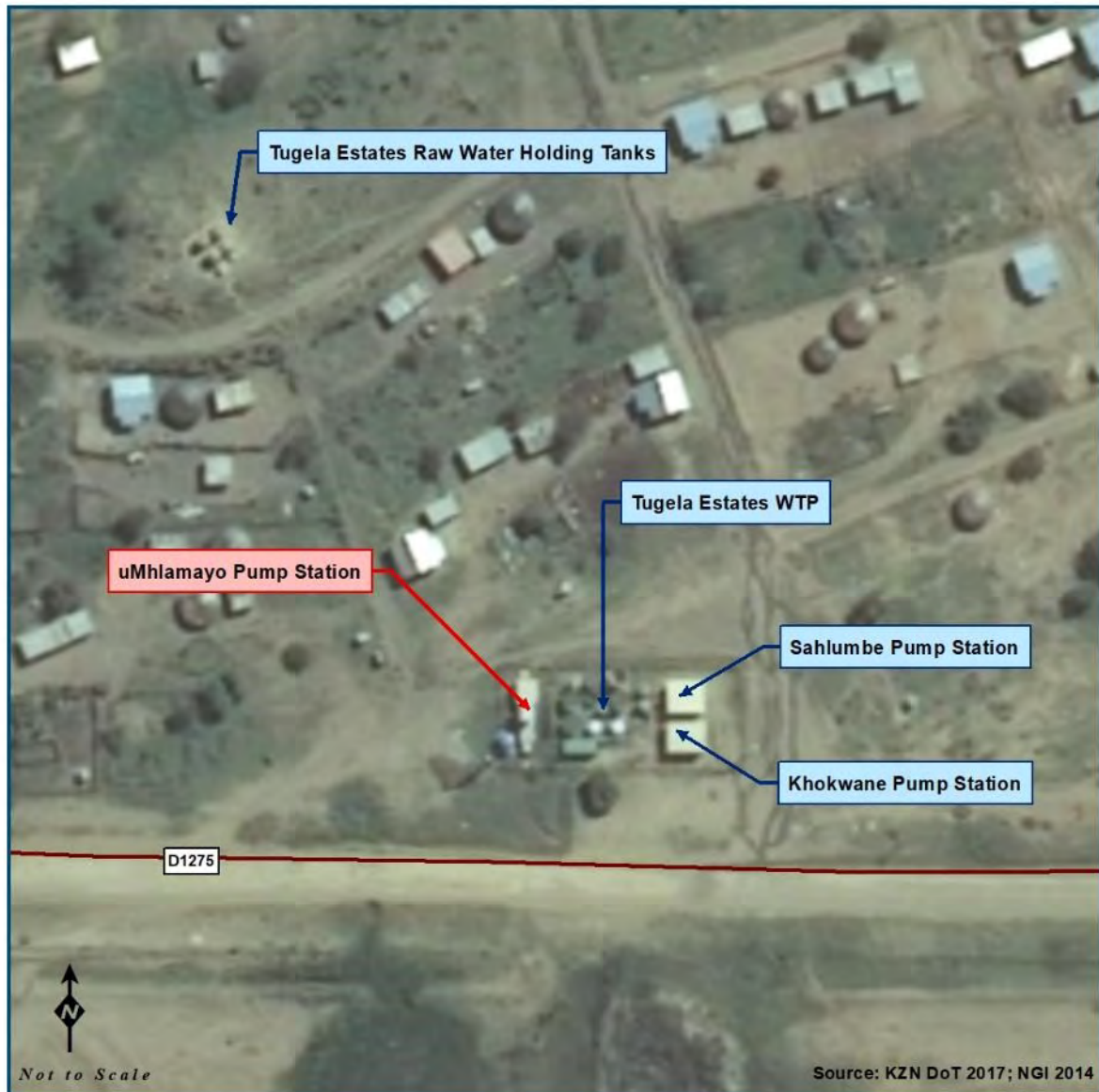
Figure 13.27 uMhlamayo Pump Station adjacent to the Tugela Estates WTP (KZN DoT 2017; NGI 2014).
