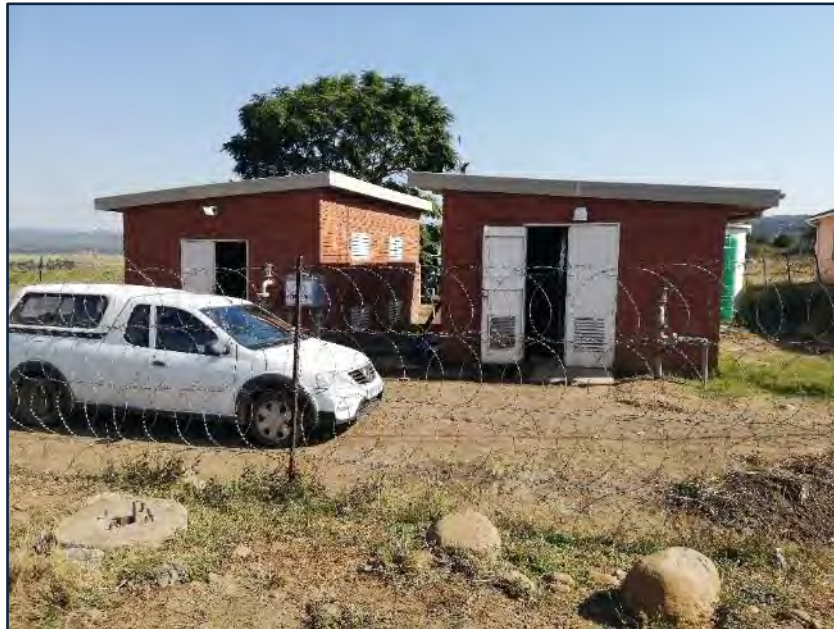
Figure 13.32 Khokwane Pump Station and Sahlumbe Pump Station on the Tugela Estates WTP site (Umgeni Water 2019).
