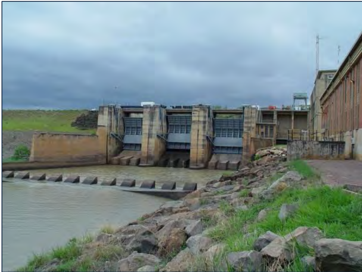
Figure 13.15 Driel Barrage Dam (DWS unknown date: DWS website).
