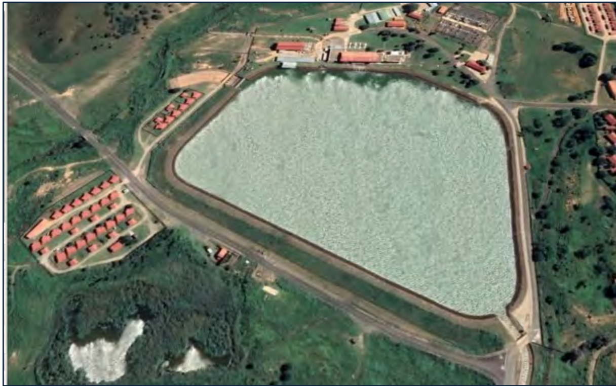
Figure 13.13 Jagersrust Balancing Dam (Google Earth 2019: website).
