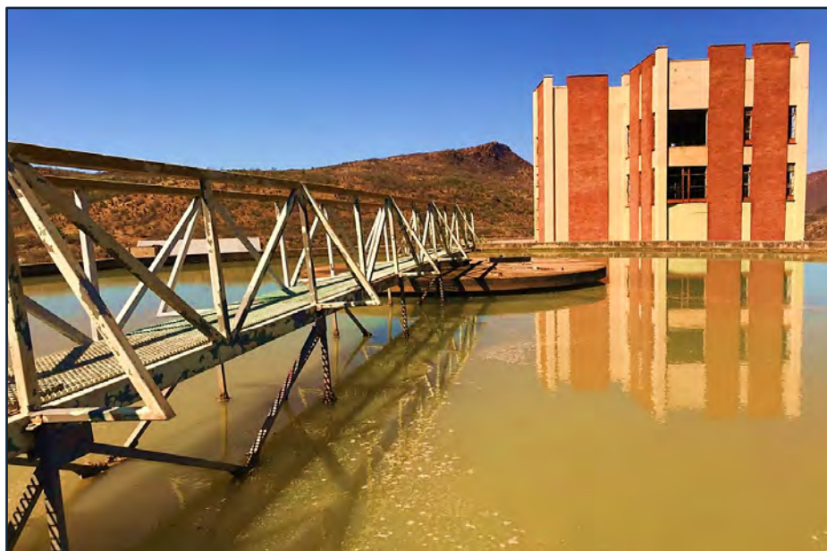
Figure 13.21 Ezakheni Water Treatment Plant (unknown date).
