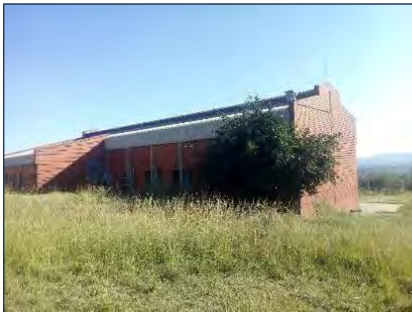
Figure 13.43 Petronella Reservoir Pump Station (Umgeni Water 2019).
