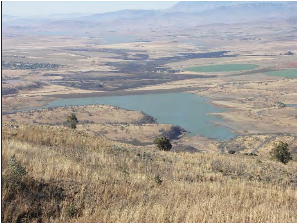
Figure 13.12 Kilburn Dam (DWS 2008: DWS website).
