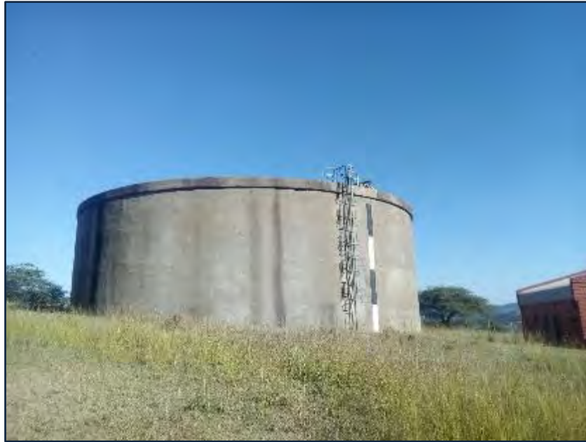
Figure 13.41 Petronella Reservoir (Umgeni Water 2019).
