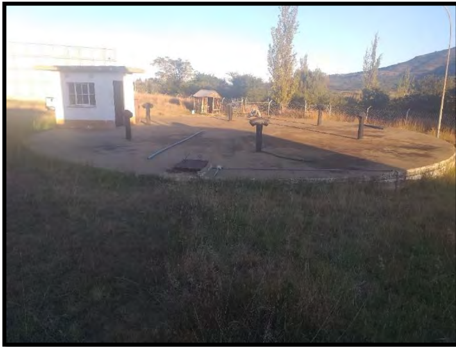
Figure 14.41 Utrecht Clear water Reservoir
