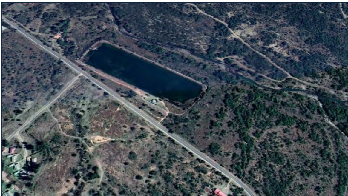
Figure 14.12 Nywersheid Dam (Google Earth 2018: website).
