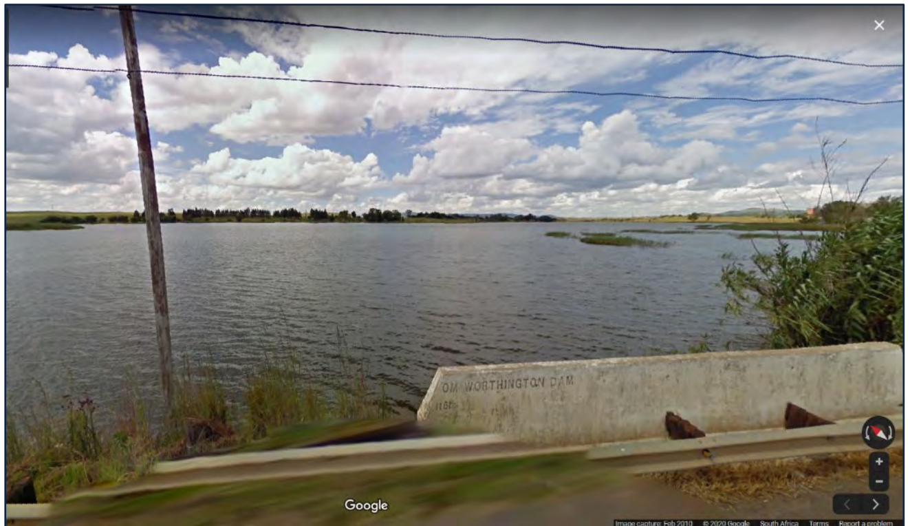
Figure 14.13 Tom Worthington Dam (Google StreetView 2010: website).
