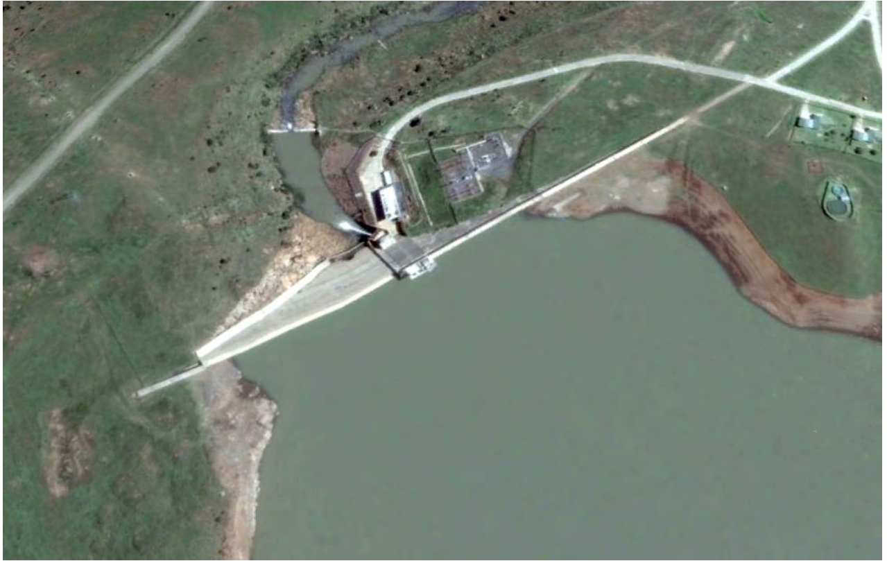
Figure 14.7 Zaaihoek Dam (Google Earth).
