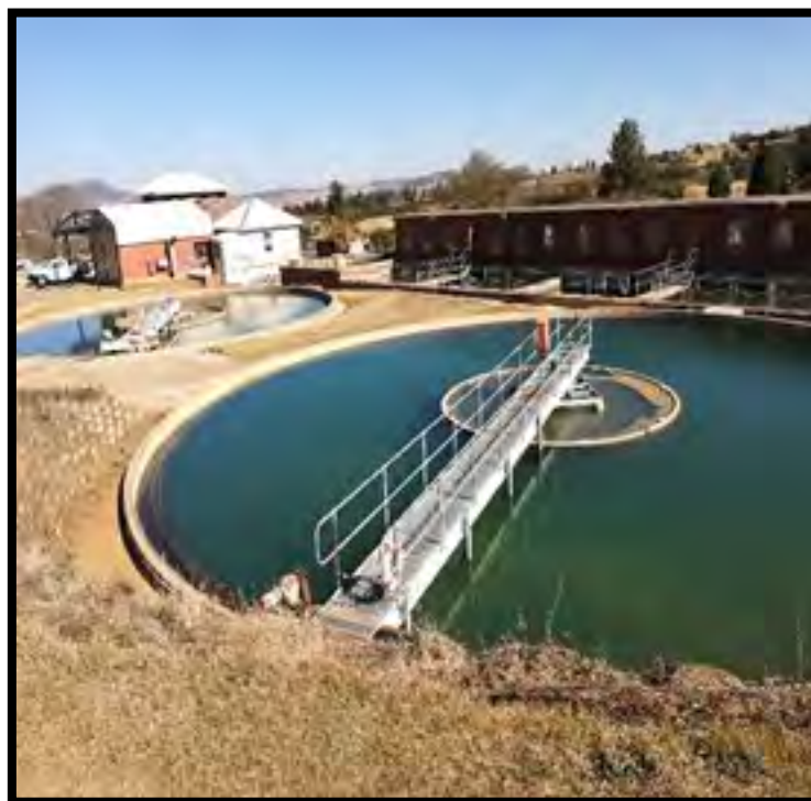
Figure 14.45 Photo of Biggarsberg WTP, Clarifiers (July 2019)
