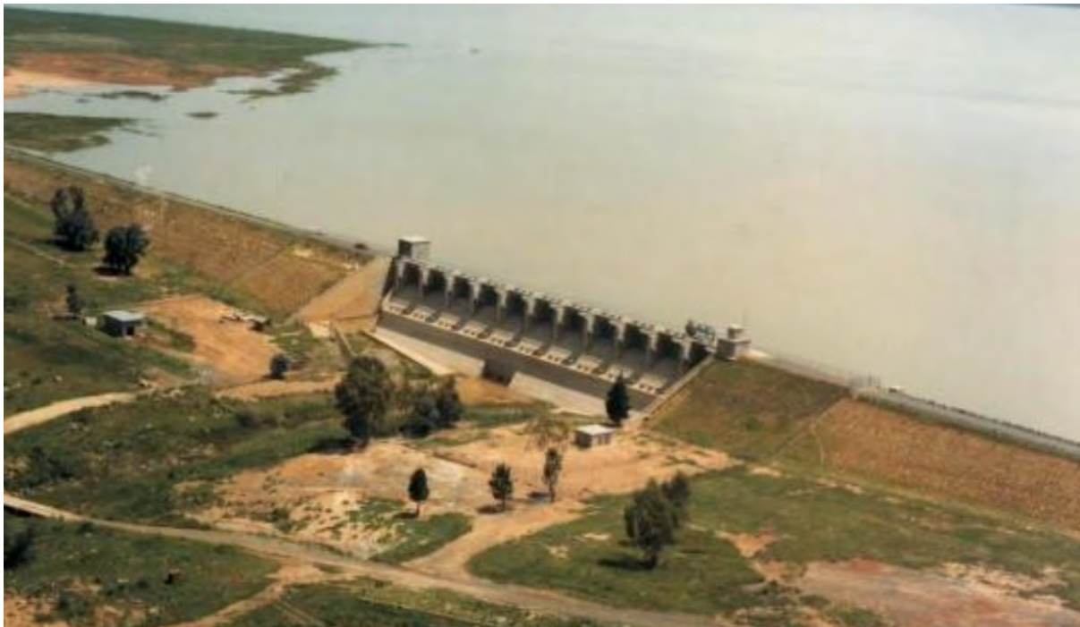
Figure 14.9 Ntshingwayo Dam (DWS 2008: DWS website).
