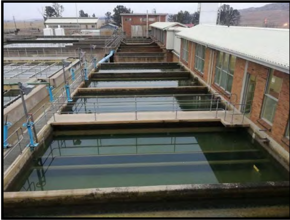
Figure 14.21 Photo of Ngagane WTP (May 2016)
