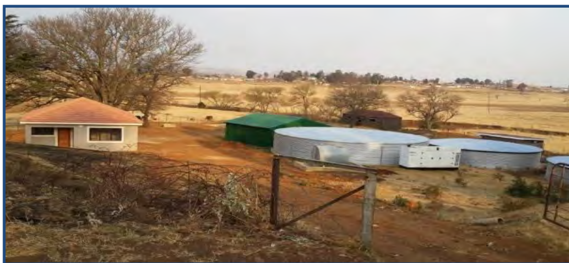
Figure 14.42 Photo of Charlestown Water Treatment Plant (July 2018).
