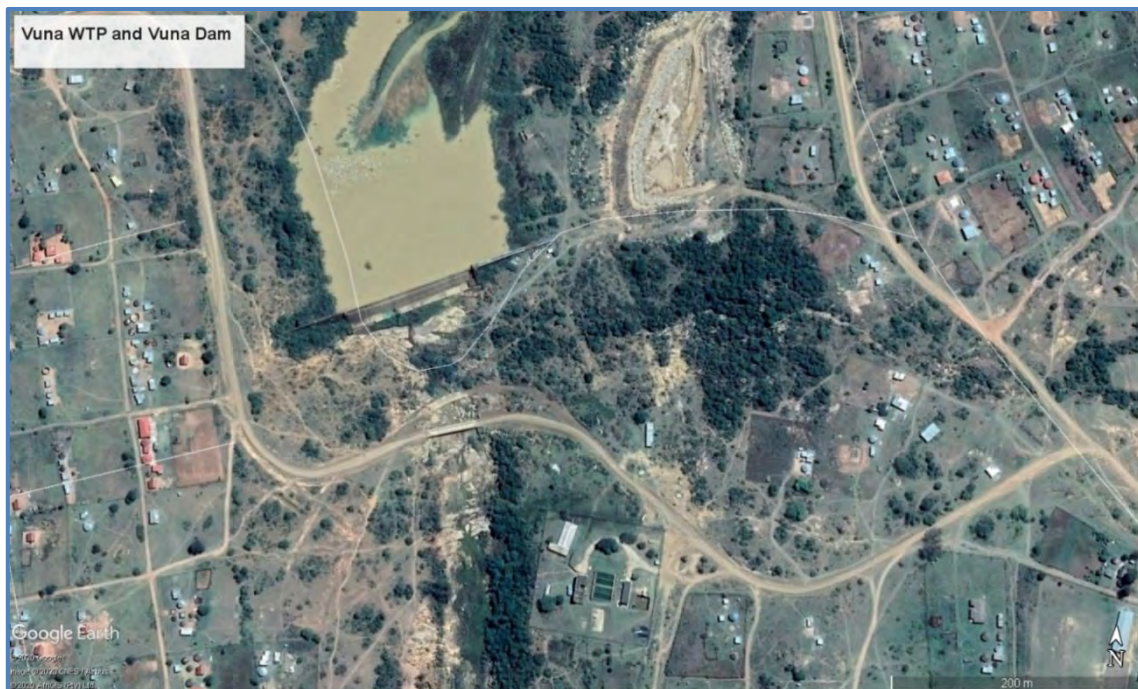
Figure 17.22 An Aerial view of the Vuna WTP and the Vuna Dam (Google Earth 2020: website).
