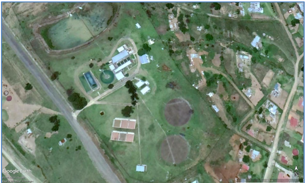
Figure 17.28 An Aerial view of the Mondlo WTP (Google Earth 2020: website).
