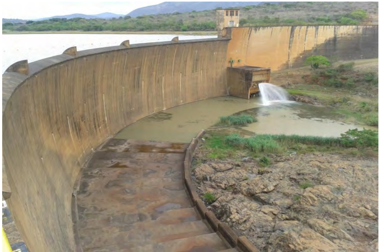
Figure 18.9 Hluhluwe Dam (DWS, 2016)
