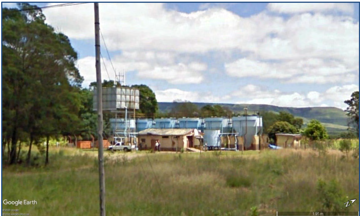
Figure 18.18 Hlobane WTP (Google Earth 2020: website).
