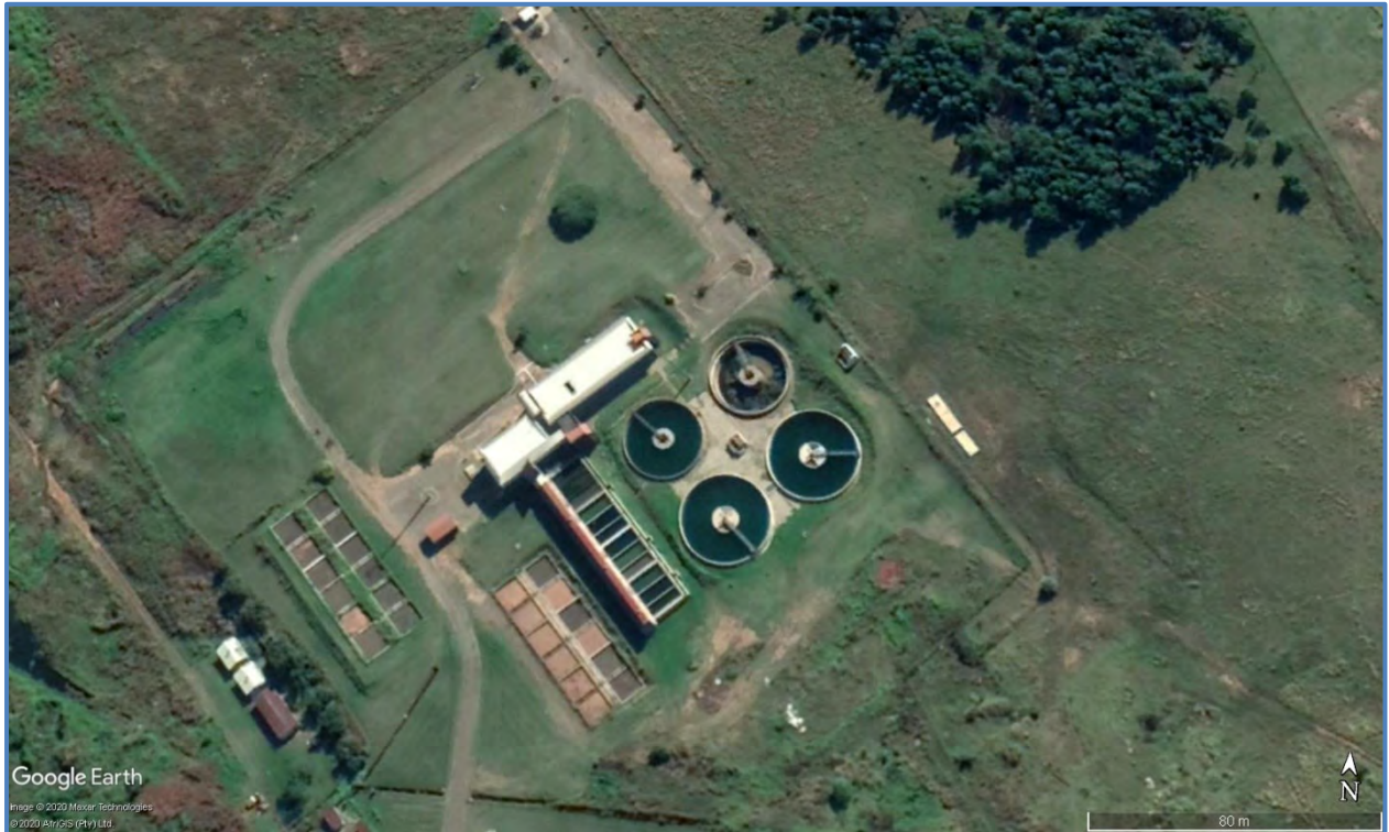
Figure 17.26 An Aerial view of the Klipfontein WTP (Google Earth 2020: website).
