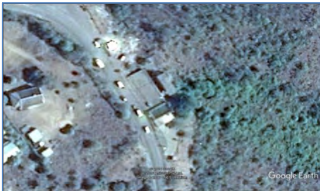
Figure 18.28 Aerial view of Jozini Old Water Treatment Plant (Google Earth 2020: website).
