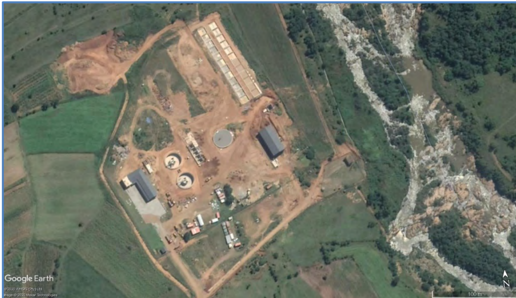
Figure 18.38 Construction of new 15 Mℓ /day WTP at Frischgewaagd along the Phongola River (Google Earth 2020: website).
