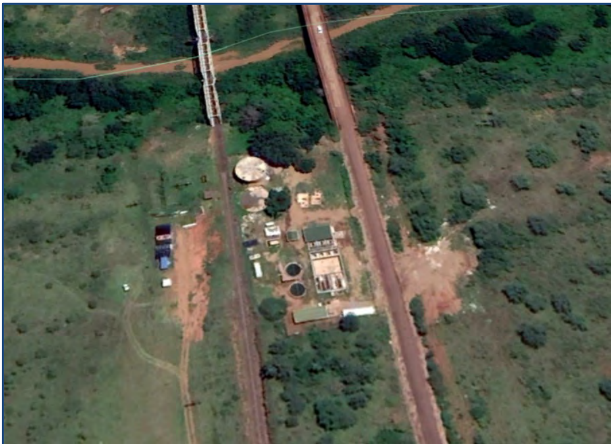
Figure 18.15 uMkhuze WTP (Google Earth 2020: website)
