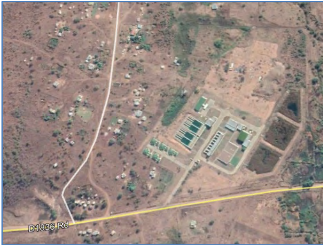
Figure 18.39 Aerial view of Regional Water Treatment Plant (NEW) (unknown source).
