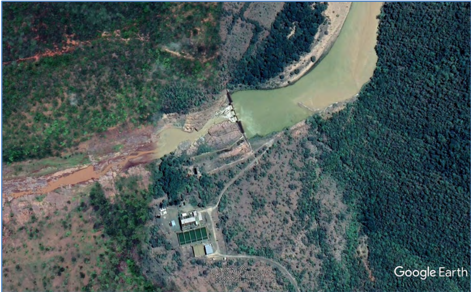
Figure 17.7 Ulundi Balancing Weir (Google Earth 2020)
