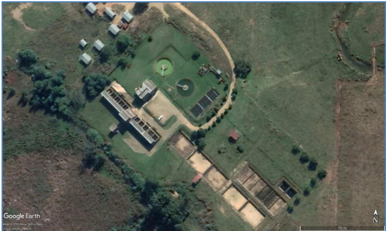
Figure 17.25 An Aerial view of the Bloemveld WTP (Google Earth 2020: website).
