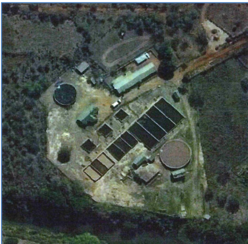
Figure 18.35 Aerial view of the Shemula (Old) WTP (unknown source).
