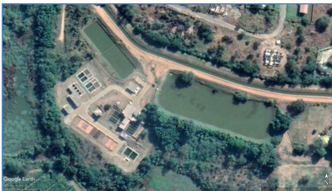
Figure 18.26 Aerial view of Phongola Water Treatment Plant
