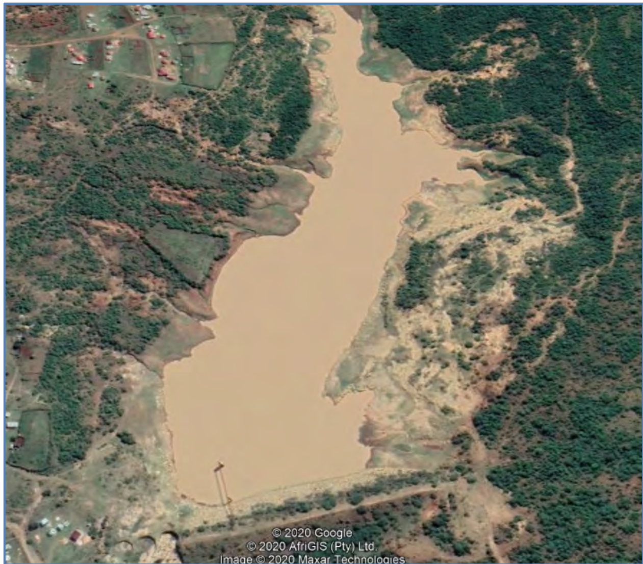
Figure 17.9 Vokwana Dam (Google Earth 2020)
