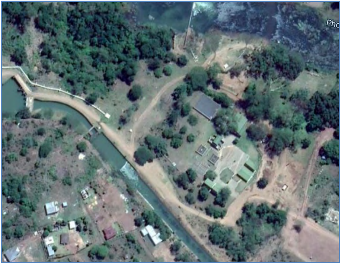
Figure 18.29 Aerial view of Jozini New Water Treatment Plant (unknown source).
